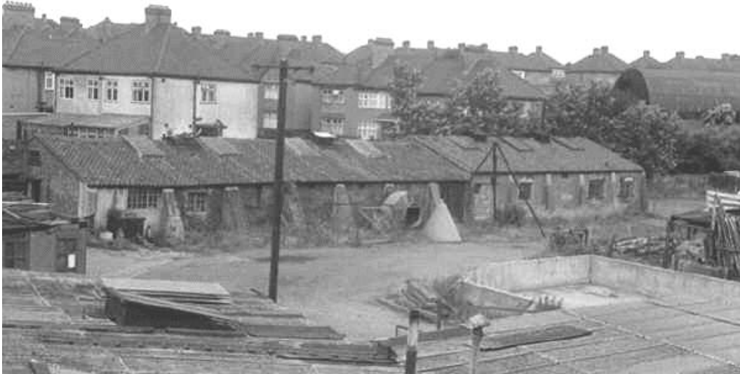
Looking north towards Norfolk Avenue – stables in mid ground
