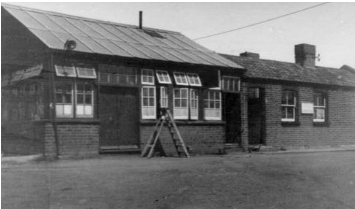
Closer view of office (right) and canteen (left)
