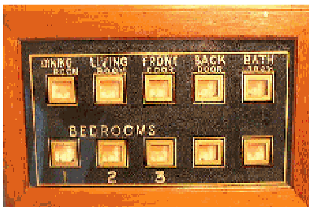
Type of indicator board installed at River House
