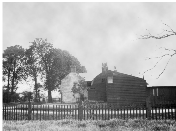
Devonshire Hill Lodge. North elevation and the lane into which victim fled (foreground) circa 1900
